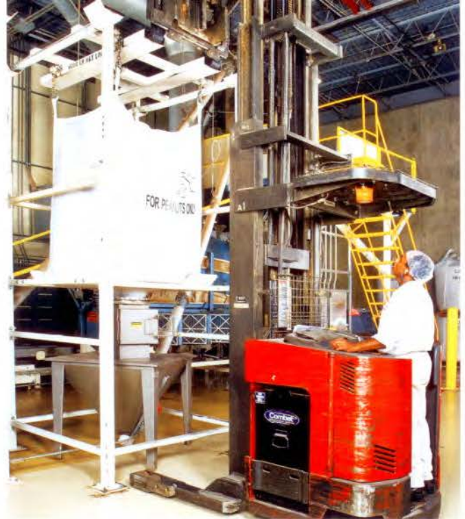
Operator forklift-loads bag-lifting frame onto the bulk bag unloader.
