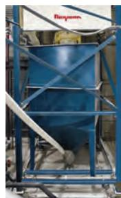
**One of two hoppers holds a 408kg bag of diatomaceous earth (DE) allowing the DE to transfer through the flexible screw conveyor to the tank**
