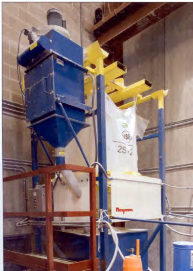
Above and Below: A Bag-Vac dust collector, mounted on the bulk bag unloader frame, vacuums displaced air and dust, and collapses empty bags dust-free prior to tie-off and removal. The bulk bag is supported in a lifting frame.
