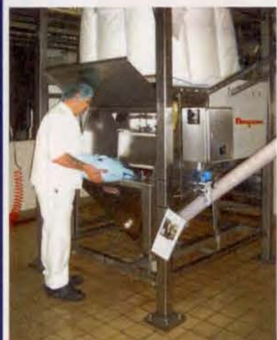
The new bulk solids handling system has contained dust and reduced injuries related to manual bag handling.
