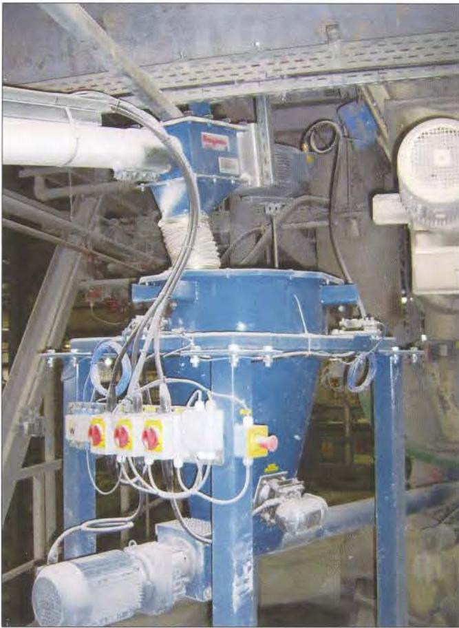
The upper flexible screw conveyor transfers aluminium powder from the bag dump station to the top of a weigh hopper, while the conveyor below feeds weighed batches to the blender.
