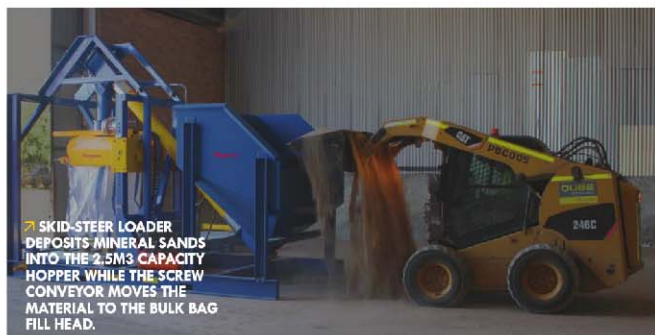
THE AUTOMATED BULK BAG FILLING STATION FILLS BULK BAGS WITH UP TO 160,000 KG OF ABRASIVE MATERIALS PER EIGHT-HOUR SHIFT
