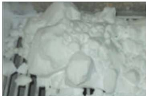
Before installing the bulk bag conditioner, manual methods to de-lump chemical powders slowed the reactor loading process.
