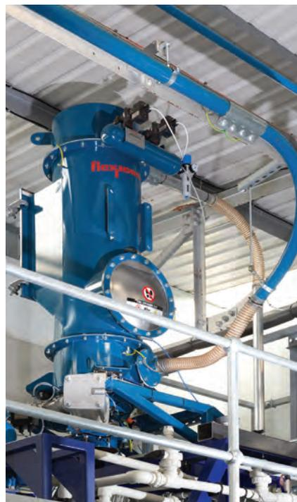
**From the pneumatic line, the filter-receiver separates the silicon powder from the air stream before the powder enters the receiving hopper and is delivered to a slurry tank. A reverse pulse jet system cleans the filter cartridges at timed intervals.**
